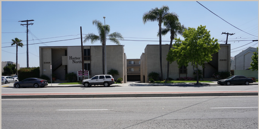
6_Multi family residential building across the street
