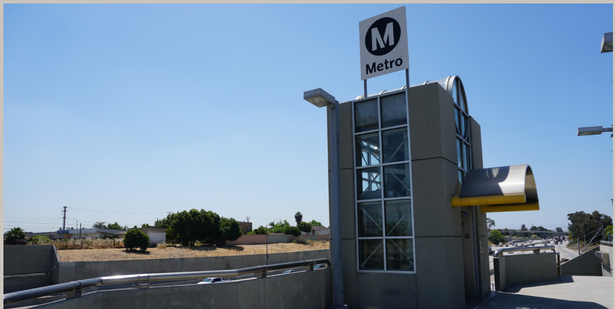
7_View of site from across the 110 Freeway at Metro Transit Center
